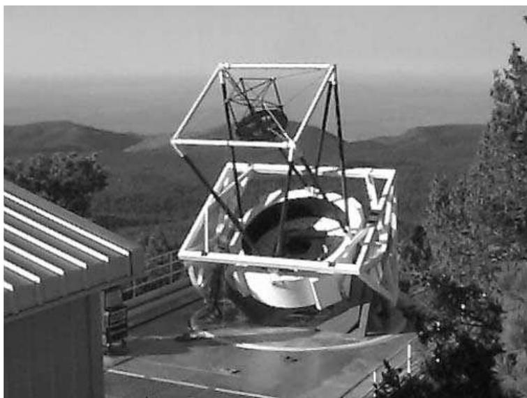
Figure 5: Photograph of the 2.5-metre telescope structure, taken shortly after installation, on 10 October 1995. Part of the telescope enclosure, in its rolled back position, appears in the bottom-left of this picture. Note that neither the mirrors nor the wind baffle are installed yet.
