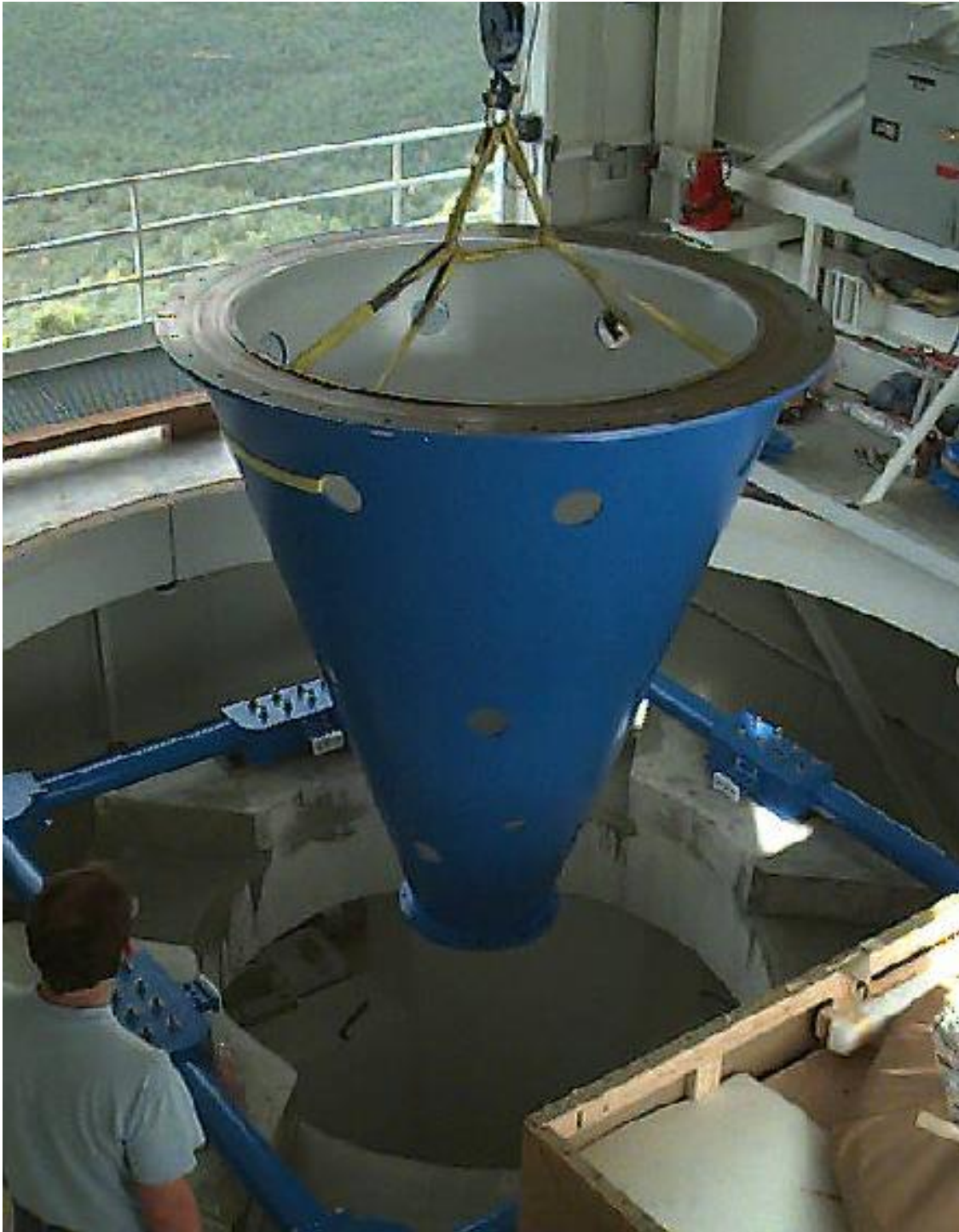
Fig. 24.— Installation of the SDSS 2.5 m telescope begins in earnest. On August 15 1995 the azimuth bearing and support is lowered into place through the floor of the support platform (see Figure 12).
