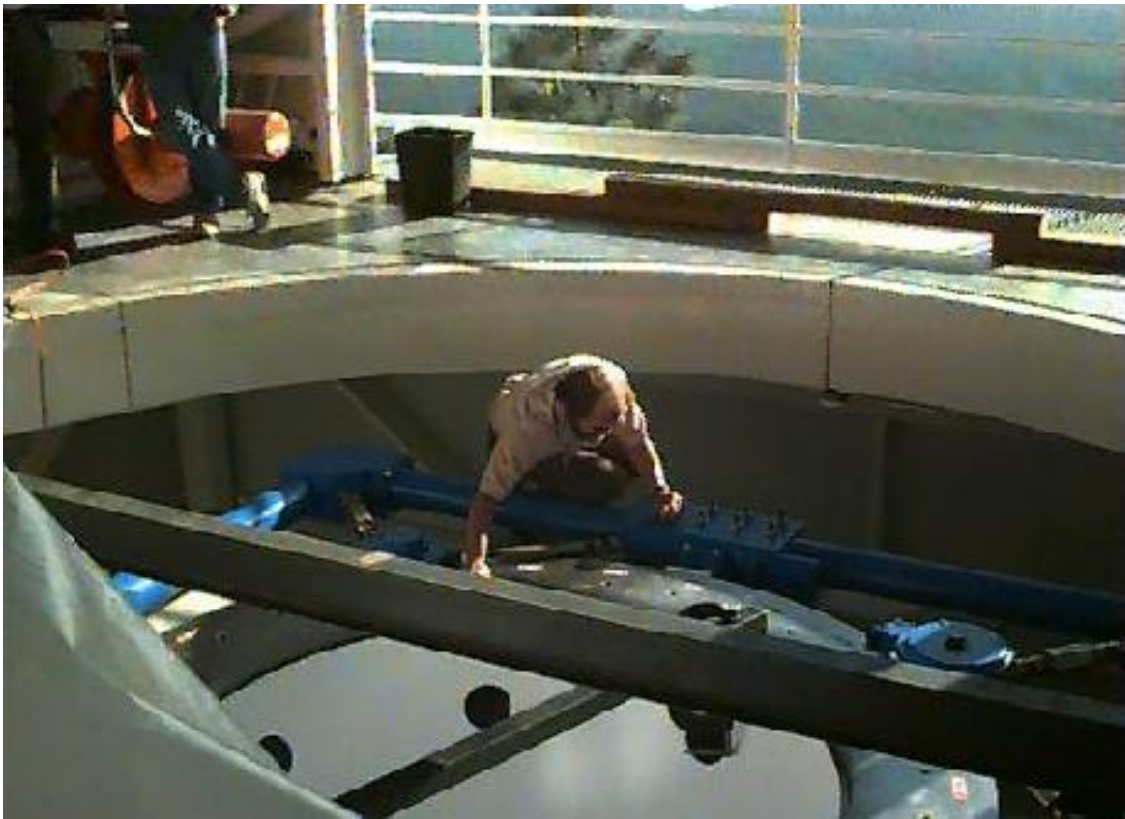
Fig. 25.— The azimuth support is installed and tested. This image shows the inspection of the azimuth drive disk.
