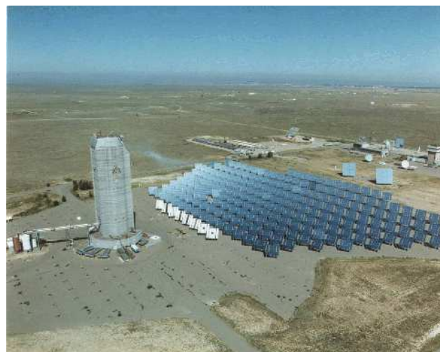
Fig. 1. Aerial view of National Solar Tower Test Facility at Sandia National Laboratories in Albuquerque, New Mexico, USA.
