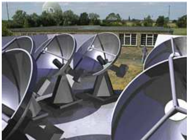
Figure 1. The Arcminute MicroKelvin Imager is planned to consist of eight 13-m dishes of the Ryle telescope, five of which are visible in the top image, and an array of 3.7-m antennas, which can be seen in the artist’s impression below.
