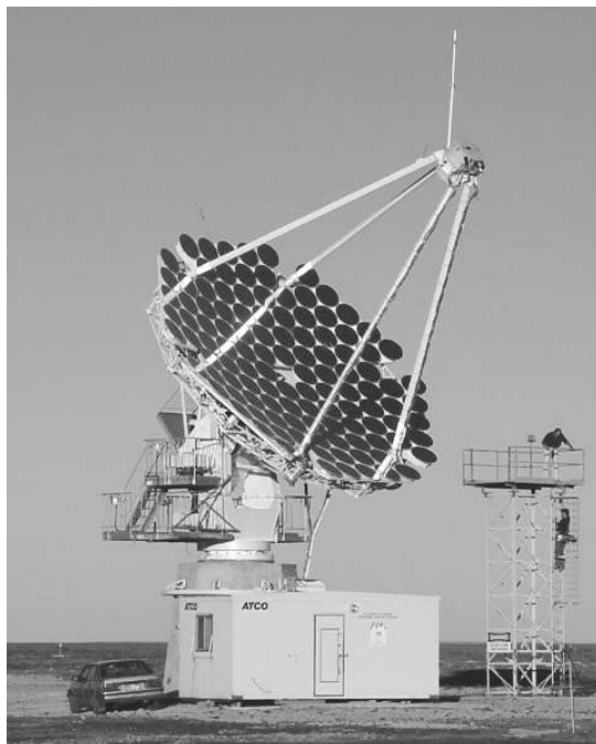
FIGURE 1. The 10 m telescope completed in February 2000 in Woomera, South Australia. The reflector consists of 114 spherical mirrors of 80 cm radius. The imaging camera is set at the focus ( f = 8 m) and can be accessed from the tower (right) for maintenance.
