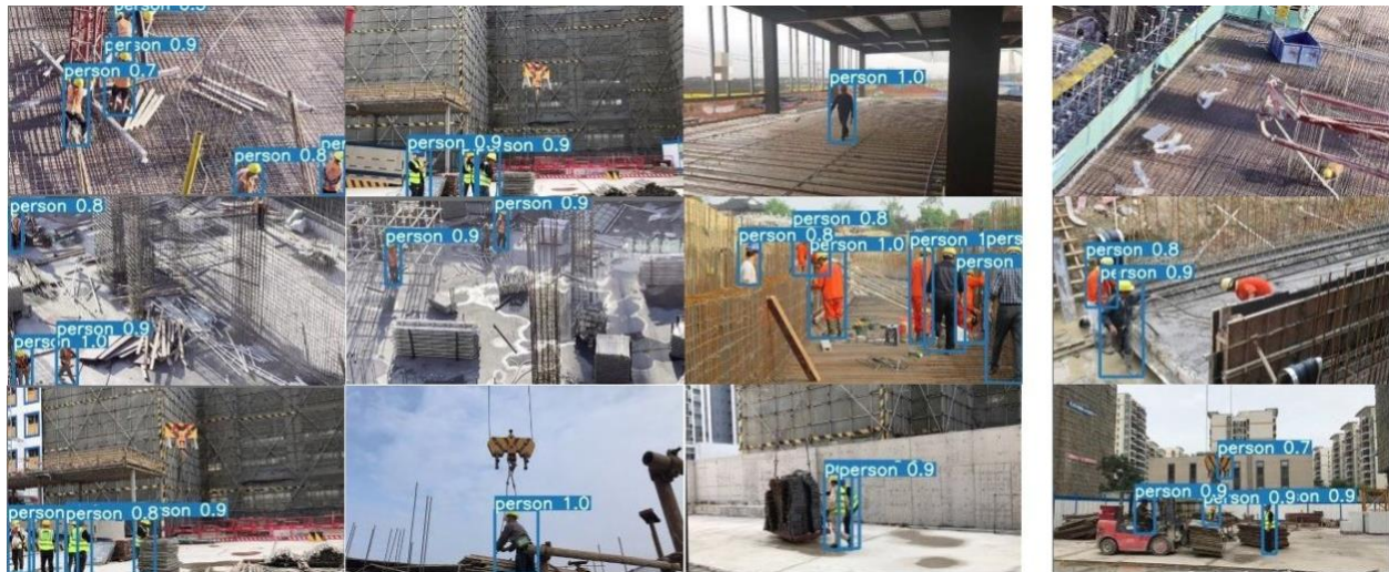
Figure 5. Performance of our model on construction worker detection. Nine successful identifications (left) and three failure cases (right) from the real test dataset are displayed.
