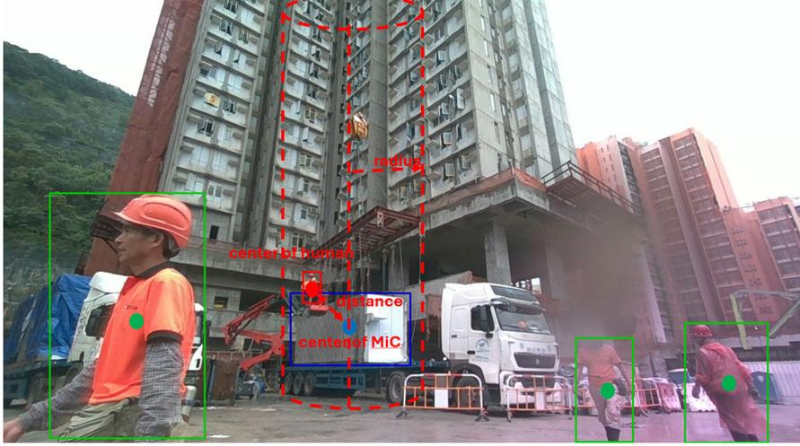
**Fig. 3** MiC lifting danger zone. The danger zone is a cylinder with radius  $r$ . The axis of the cylinder pass through the center of the MiC and is perpendicular to the ground.
