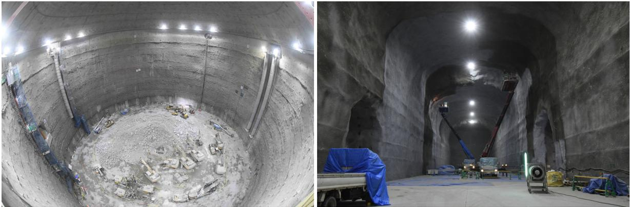
Figure 1: Photographs of the Hyper-K cavern during the excavation in September 2024. Left: the main cavern being excavated to a depth of 45 m in the barrel section. Right: the water purification system room under dust-proof coating.
