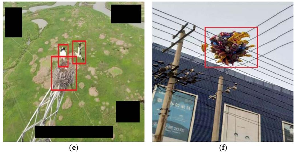
**Figure 1.** Collection of Foreign Object Image Datasets for Transmission Lines. (a) trash. (b) twig. (c) nest. (d) kite. (e) bird. (f) balloon.
