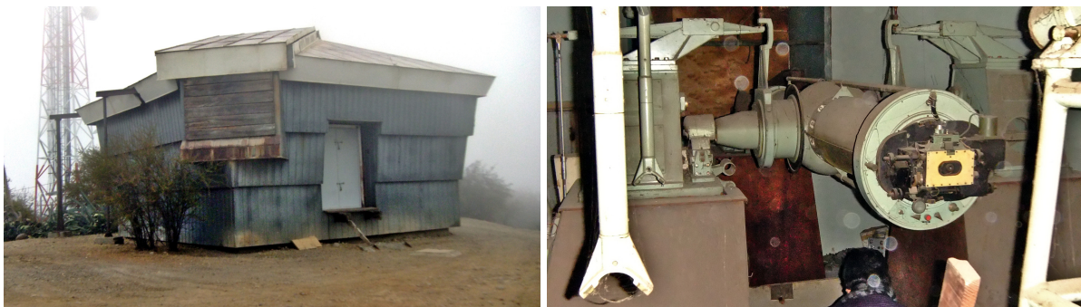
Figure 11. The rhomboidal-shape dome designed by Yu.S. Streletsky for the Pulkovo large transit instrument at the Cerro Calan observatory (Chile) in the 1960s and the large transit instrument inside (photos by the author, 2013).
