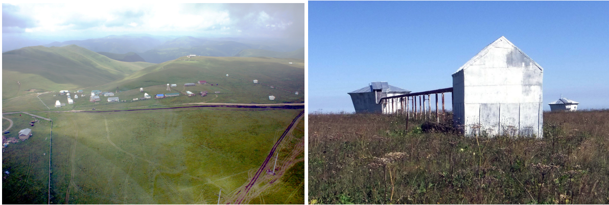
Figure 10. Kislovodsk Mountain Station of Pulkovo Observatory (left) where two Ertel-Struve classical instruments, the vertical circle and the large transit instrument were installed during 1984 to 1989 in the rhomboidal-shape domes (right) designed by Yu.S. Streletsky. One of the domes is equipped with two meridian marks for monitoring the transit instrument's azimuth (photos by the author, 2012).
