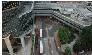
The pedestrians between the bus stop and white bus.
