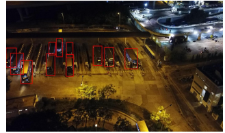
The buses parked in rows within the depot.
