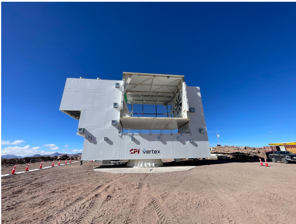
Figure 10. A photo of the LAT at the Chilean site, as of March 2024. In this image, the receiver cabin is located towards the top left of the structure.
