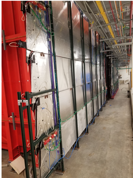
Figure 15: The Side CRT East walls post-installation.
