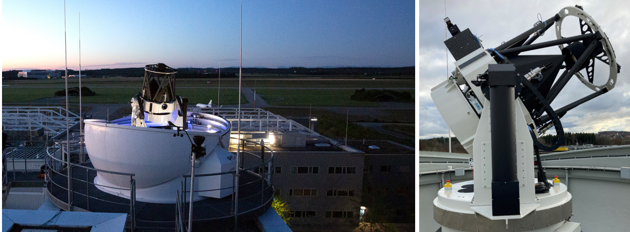
Fig. 4. The left panel shows the OGS-OP NG on the rooftop of DLR-IKN in Oberpfaffenhofen, southern Bavaria, Germany. The right panel zooms in onto the 80 cm Nasmyth-Design telescope.
