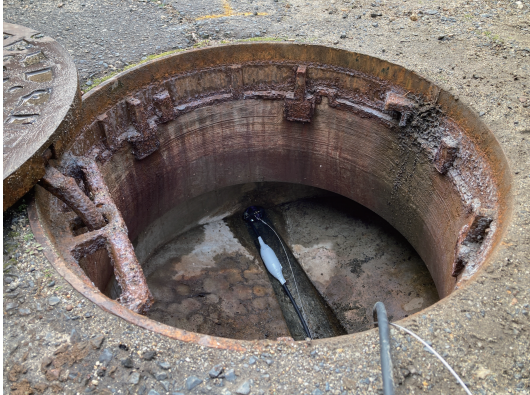
Fig. 13. AIRo-7.1 entering a force main in sewer pipes.
