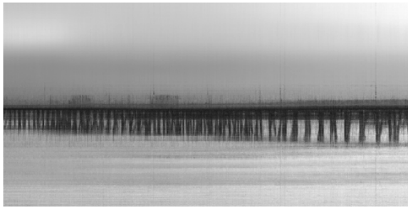
Bridge restored with NN.
