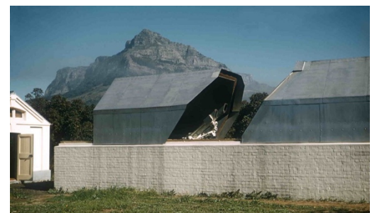
Fig 6: The Lyot Coronagraph In better days. This telescope followed the Sun automatically from dawn to sunset. The H\alpha filter was thermostatically controlled.
