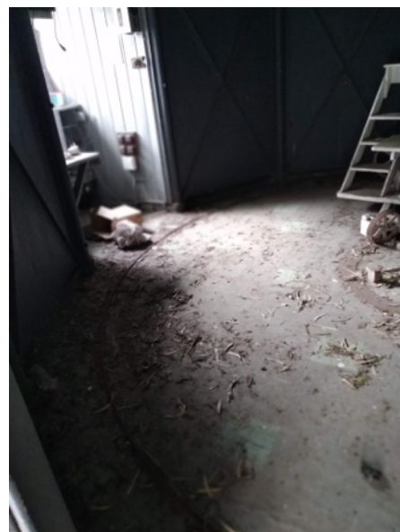
Fig 20: The building has been invaded by starlings and the floor is covered by straw and bird droppings.
