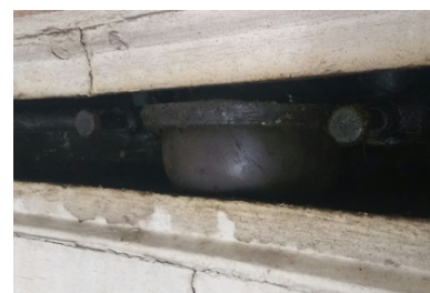
Fig 25: One of the cannon ball “bearings” of the dome.
