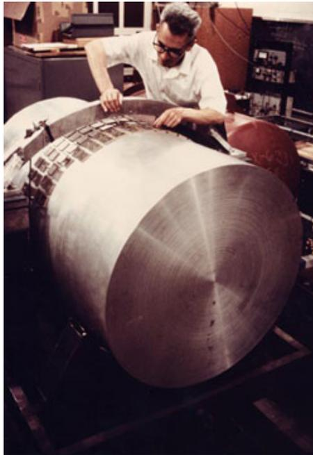
Fig. 1. Weber is adjusting the instrumentation: one of his aluminum cylinders, 2 meters in length and 1 meter in diameter, for detecting gravitational waves. [Image Credit: <https://physics.aps.org/story/v16/st19>]
