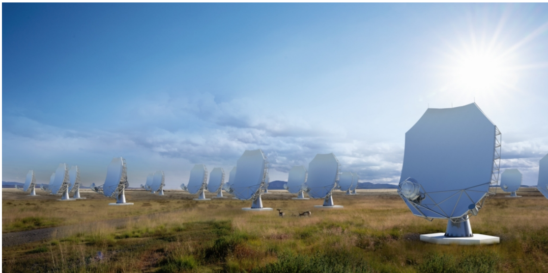
Figure 1: Artist's conception of the mtex design for the ngVLA prototype antenna (credit: Sophia Dagnello, NRAO/AUI/NSF). The array will consist of three components: a main interferometric array with 214 \times 18 m reflector antennas covering baselines up to 1068 km, a short baseline array with 19 \times 6 m antennas covering the shortest baselines, and a long baseline array with 30 \times 18 m antennas covering baselines up to 8860 km. It will be deployed in the southern US and northern Mexico, with long baselines reaching up to Canada and down to Puerto Rico and the US Virgin Islands. This will be sufficient to achieve sub-milliarcsecond resolution. The array will operate between wavelengths of 21 cm and 3 mm.
