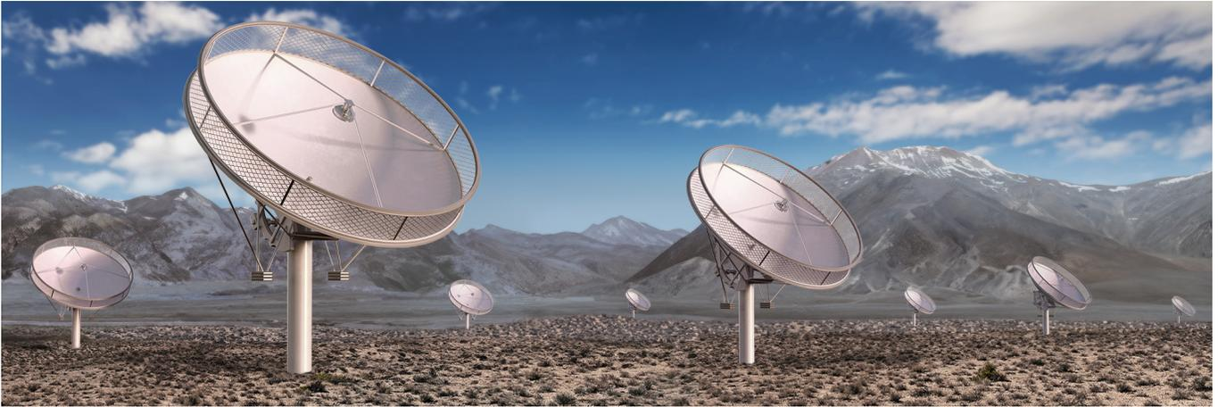
**Figure 1.** Artist’s rendering of the DSA-2000 antennas. Each dish has a diameter of 5 m, and the antennas are fully steerable in azimuth and elevation. The array will consist of approximately 2000 such antennas, configured as pictured in Figure 2.
