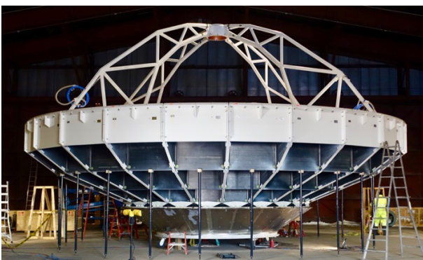
Figure 2. The backup structure is shown after the assembly of the carbon fiber segments and quadrupod on the invar cone in one of the hangars of the PAB.
