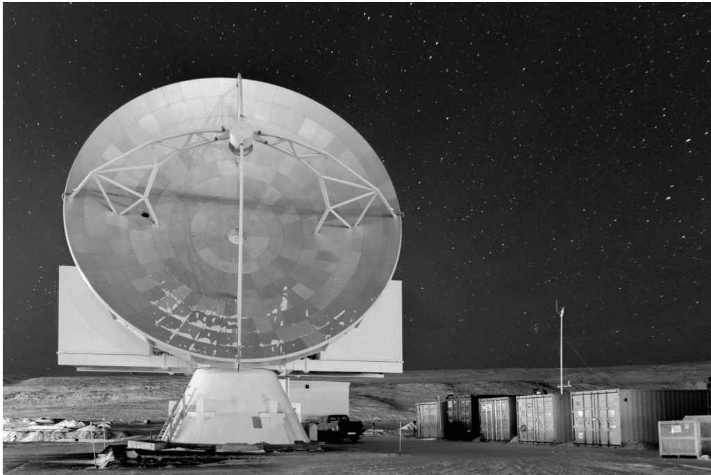
Figure 3. The GLT under commissioning in PSB [10]. The newly added side-containers are partially seen behind the primary dish. The containers shown in the lower right corner of the photo are our working spaces and storage facilities. Some snow can be seen in the lower part of the primary dish. At that moment, the de-ice system was not yet implemented. The hole on the left side of the dish, near the base of the quadrupod, is the location of the optical guide scope.
