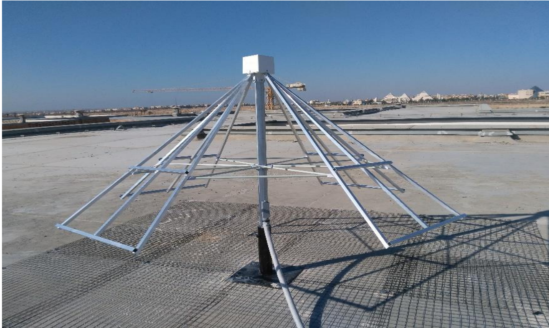
Fig. 1: Installed long-wavelength array antenna on the top of the Space Environment Research Lab-EJUST building at N30°, E29°. The antenna is an aluminum frame with a CDA, active balun, and ground screen made of a steel grid with a cell size of 2.47 mm x 2.47 mm.
