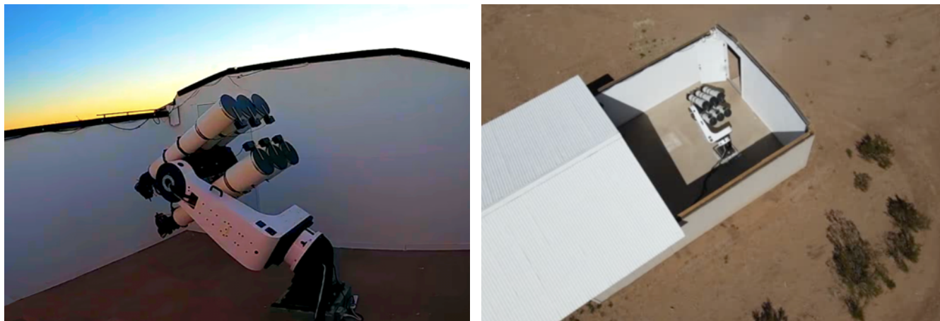
Figure 2. Images of Condor in its observatory building with a roll-off roof at the Dark Sky New Mexico observatory near Animas, New Mexico. In both images, the dust covers are closed.
