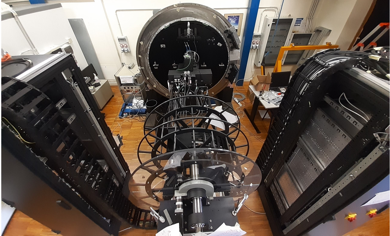
Figure 3. The corotator system includes two cable-chains routing the cables from the two electronic cabinets to the instrument.
