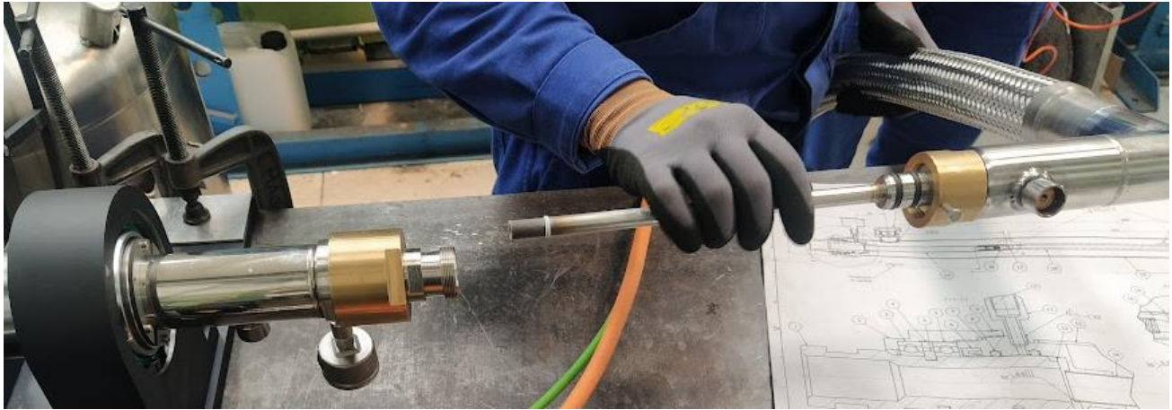
Figure 22. Installation of the flexible line on the rotating joint.
