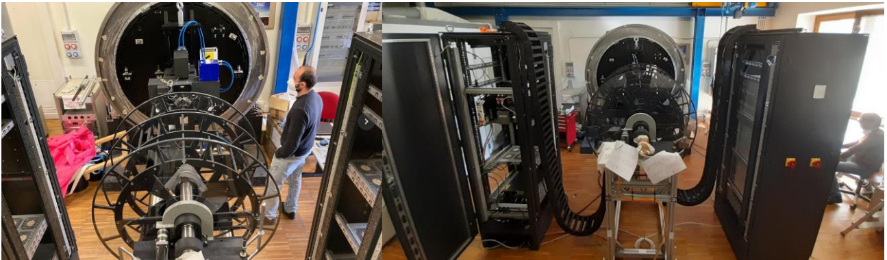
Figure 29. Left: installation of the cabinets. Right: installation of the flexible rails.
