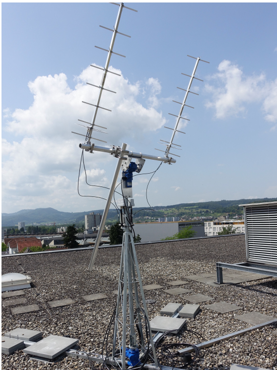
Figure 4: Switzerland UHF ground station at the campus of FHNW in Windisch.
