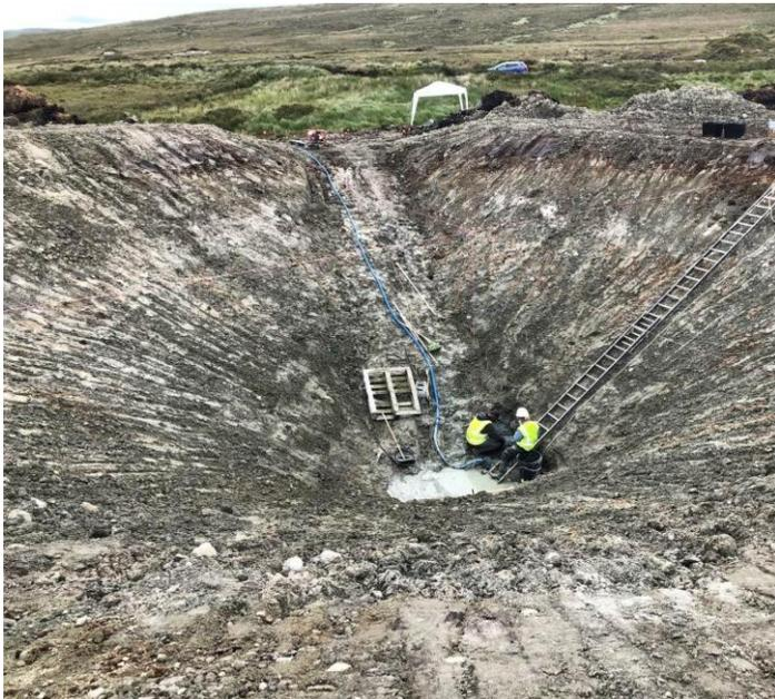
**Figure A2.** Excavation in 2019 to depth of 5.7 m and showing access ramp, submersible water pump and hose, and exit ladder. Examining the bottom and recovering rock fragments had to be done by feel at this stage.
