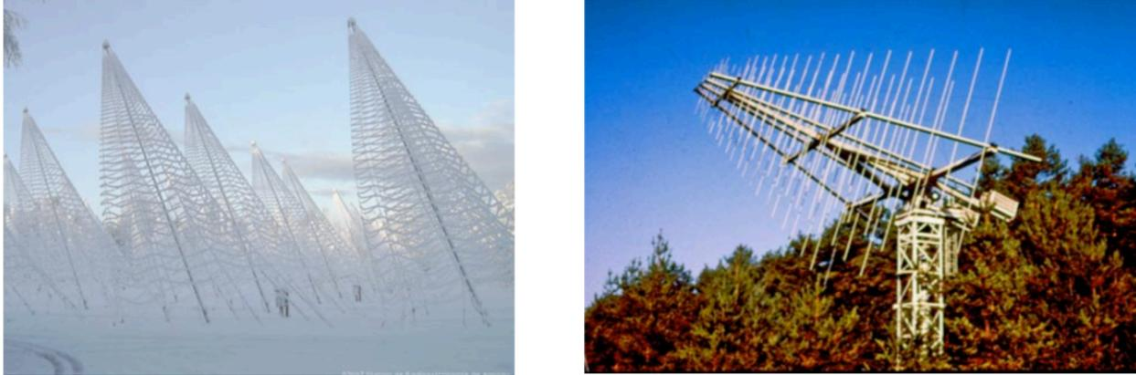
Figure 1. (Left) The Nançay Decameter Array consists in 144 helicoidal antennae divided in two left-handed and right-handed polarized subsets [1]. (Right) Historic log-periodic Yagi antenna in Nançay [2].
