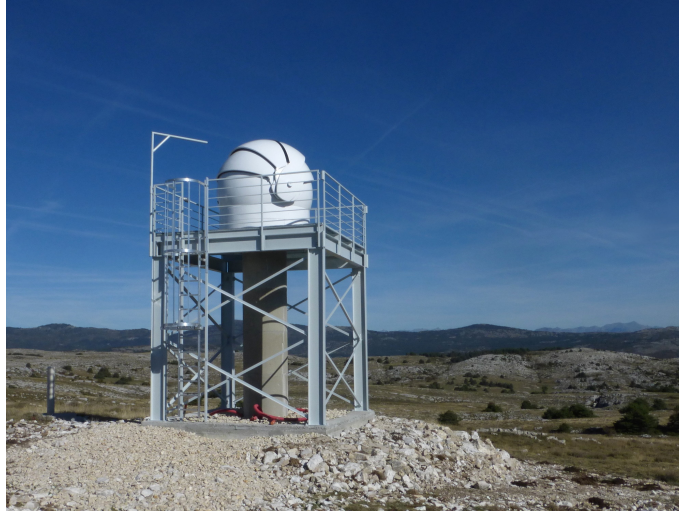
Figure 1: The GDIMM tower just after its installation on the Plateau de Calern in September 2015
