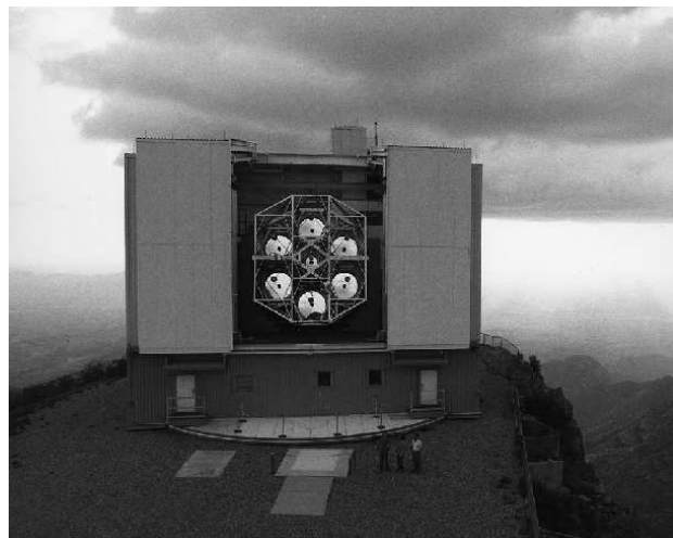
Fig. 3 The original Multiple Mirror Telescope on Mount Hopkins, Arizona, consisting of six 1.8-m mirrors in a common mount and with a common focus. Photo: Smithsonian Institution Archives.
