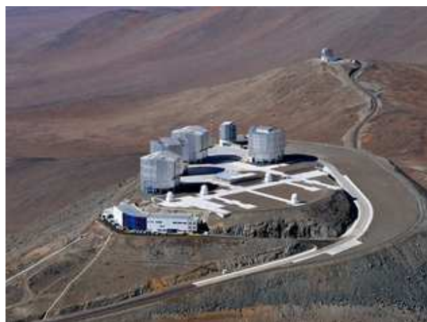
Fig. 6 The Very Large Telescope (VLT) of the European Southern Observatory at Paranal, Chile. The light from the four large (8.2-m) telescopes and the four smaller (1.8-m) telescopes can be combined coherently to reach an angular resolution at visual/NIR wavelengths of about one milliarc-second. (Credit: ESO).
