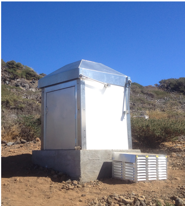
Fig. 1. The northern MASCARA station on La Palma (Spain). The box next to the station contains the heat exchanger used in the decommissioned liquid cooling system.
