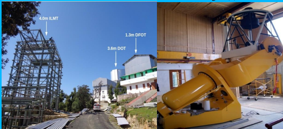
Fig. 8 (a) Devasthal Observatory showing location of all three telescopes and (b) Mechanical structure of the 1.3m telescope within a sliding dome
