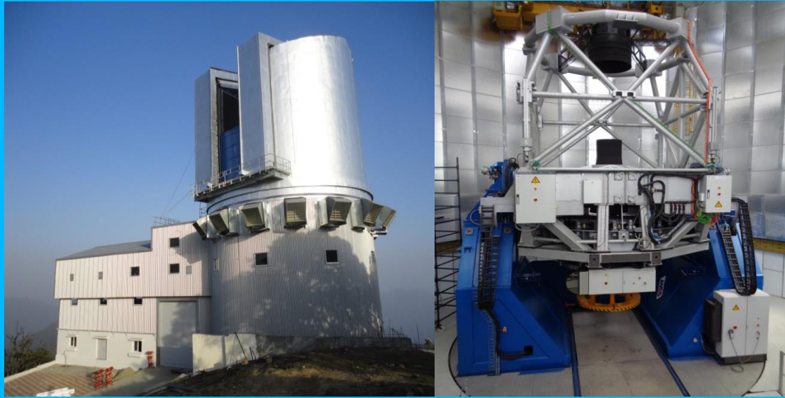
Fig. 9 (a) Building of the 3.6 meter telescope and (b) A fully assembled 3.6m DOT in its dome at Devasthal
