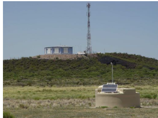
Figure B.3: A fluorescence telescope enclosure, seen on the hill top, and a surface detector station, below.
