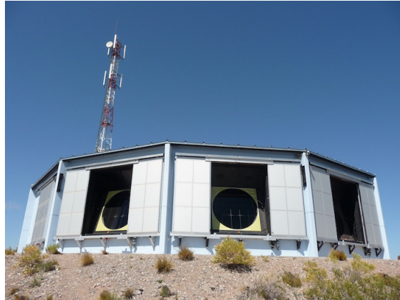
Figure B.6: FD building at Los Leones during the day. Behind the building is a communication tower. This photo was taken during daytime when shutters were opened because of maintenance.
