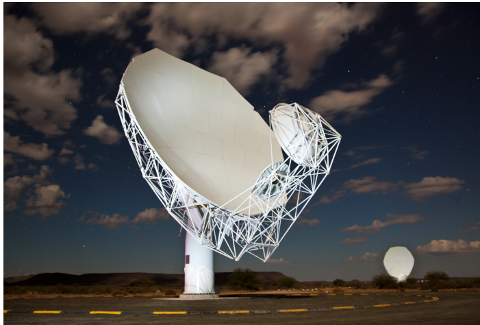
Figure 2. A MeerKAT antenna with its offset Gregorian feed.
