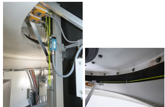
Figure 6. Photos of the Azimuth Emergency limit switch arrangement. The left photo shows the pulley arrangement, and the right photo is the cord payout around the inside of the cable wrap room ceiling. Also in the second image on the left hand side can be seen the new mounting position of the Azimuth limit switch. (Images courtesy of Stuart Weston)
