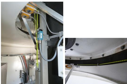
**Figure 5.** Photos of azimuth emergency limit switch arrangement. On the left is the pulley arrangement, and on the right is the cord play-out around the inside of the cable wrap room ceiling. Images courtesy of Stuart Weston
