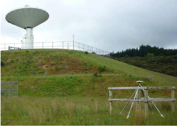
Figure 14. Collocated space geodesy facilities: the GNSS base station at Warkworth (WARK) and the IVS network station WARK12M (12m radio telescope). (Image courtesy of Sergei Gulyaev)
