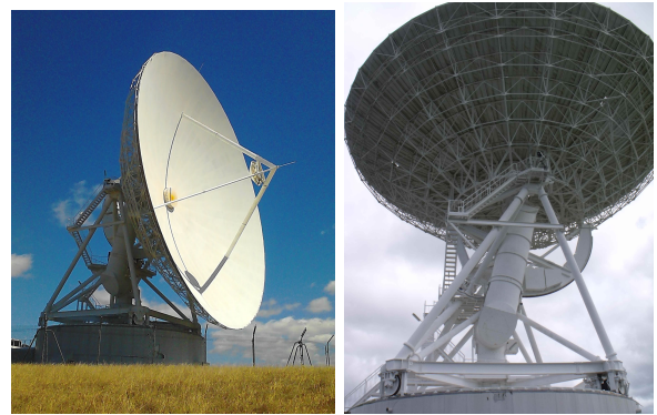
Figure 3. Photographs of the 30-m antenna after cleaning. (Images courtesy of Stuart Weston)
