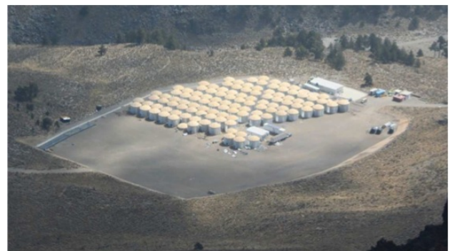
Figure 4: The High Altitude Water Cherenkov (HAWC) observatory on the Pico de Orizaba, with 100 tanks installed (one-third of the completed detector)
