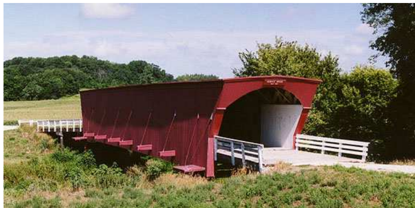
Figure 8: One of the covered bridges of Iowa.
