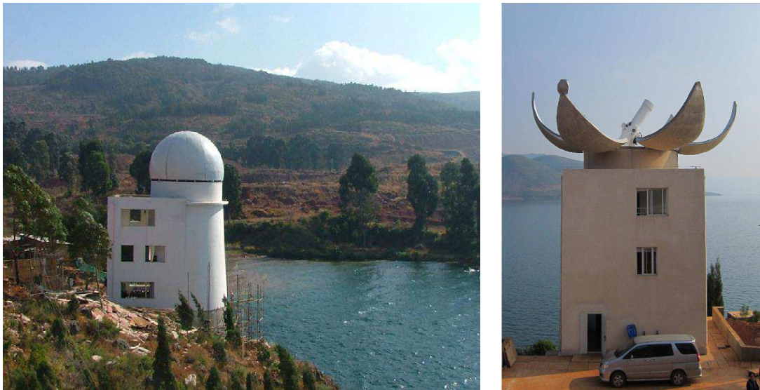
Fig. 1 The ONSET building near Fuxian Lake ( left ) and the telescope inside the blossom dome ( right ). The left picture was taken during the construction of the building.
