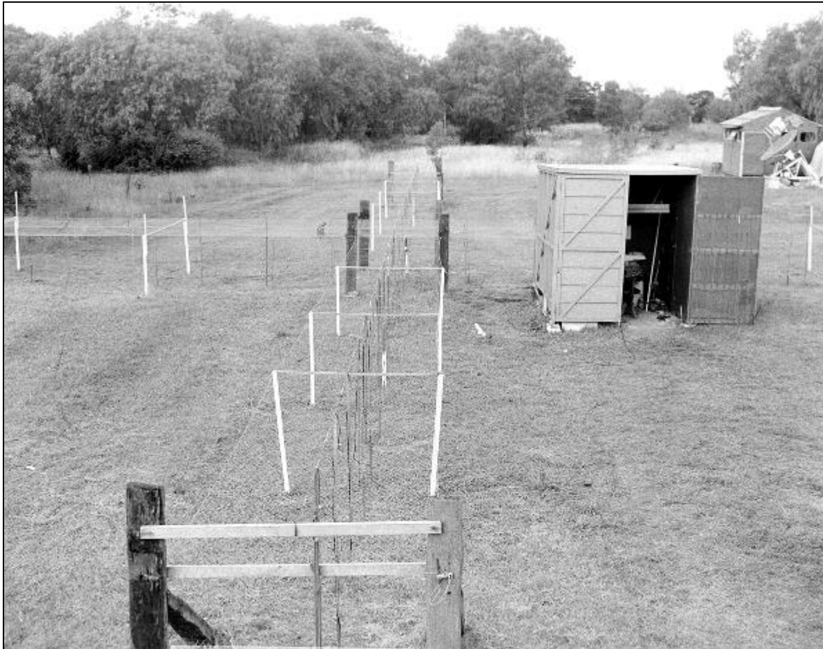
Figure 3: A close up view of the prototype Mills Cross at the Potts Hill field station. The prototype cross operated at 97 MHz with a beamwidth of 8 degrees. Each arm of the cross was 36m in length (Courtesy of CSIRO Radio Astronomy Image Archive: B3064-3 Image Date: 21 April 1953).
