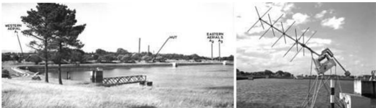
Figure 1: Potts Hill field station and the swept-lobe interferometer used by Mills for observations of Cygnus A. The left figure shows the location of the three aerials of the swept-lobe interferometer and the associated receiver hut. The view is looking to the northeast. The right figure shows a close up view of the western Yagi aerial (Courtesy of the CSIRO Radio Astronomy Image Archive: 2312 & 2217 Image Date: 28 July 1950).
