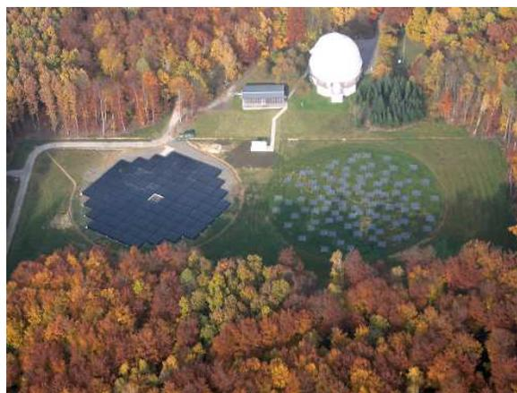
**Fig. 3** International LOFAR station near Tautenburg/Germany. Front left: dense array of dipole “tiles” for frequencies of 110–240 MHz; front right: sparse dipole array for 10–80 MHz; back: optical Schmidt telescope (copyright: Michael Pluto, Thüringer Landessternwarte).
