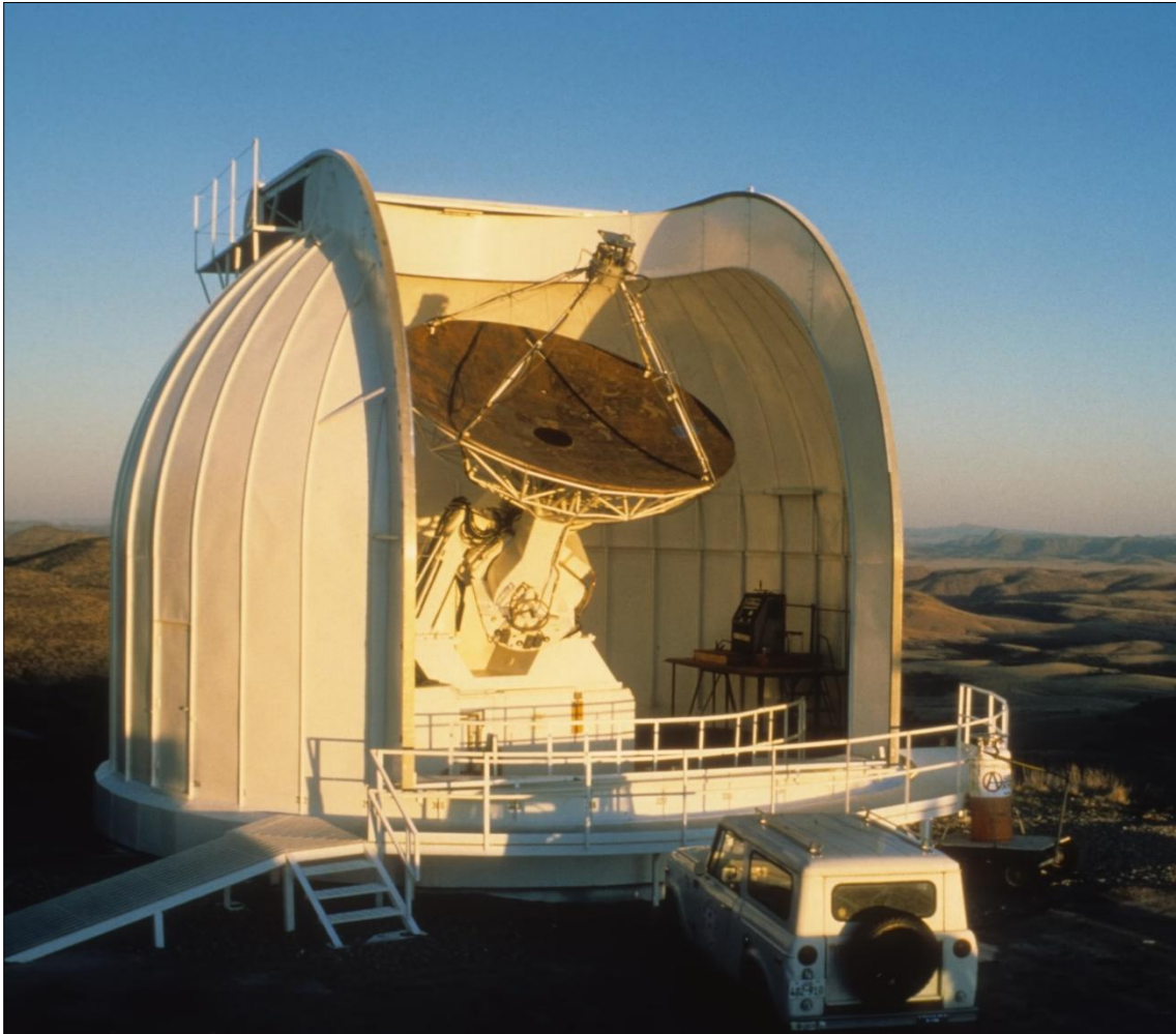
Figure 3: Photograph of the MWO 4.9-meter antenna and astrodome following dome renovations and installation of the error-correcting subreflector and high-frequency receiver box (courtesy: McDonald Observatory).
