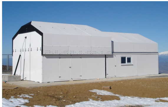
Fig. 12.— TFRM reinforced glass-fiber enclosure installed at OAdM, with sliding roof and South gabling wall.
