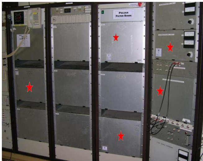
FIG. 5.— Some of the racks of the Parkes old control room. The red stars mark various pieces of hardware, including parts of the 21-cm analogue filterbank, built at the Bologna Astronomical Observatory and the IRA-Medicina radio telescope (Italy).
