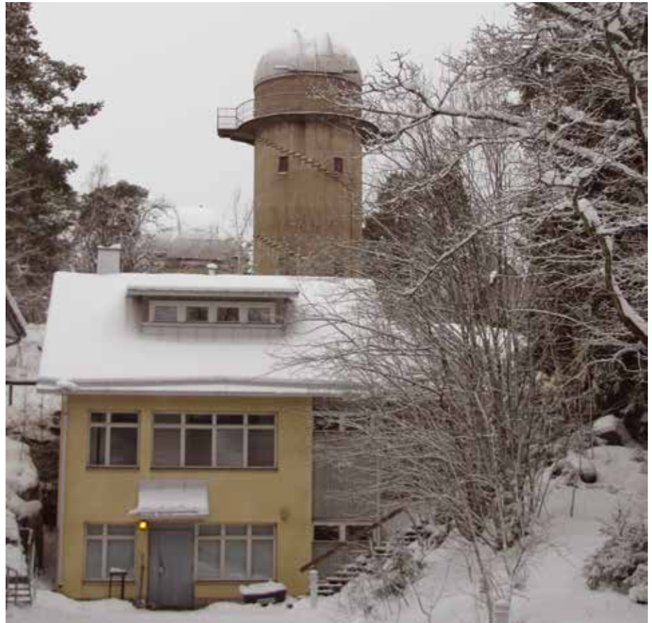
The one-metre telescope of the Tuorla Observatory in Finland is mounted on a high tower to raise it above the level of the surrounding forest. Tuorla is operated by the University of Turku, and is the largest astronomical research institute in the country.
