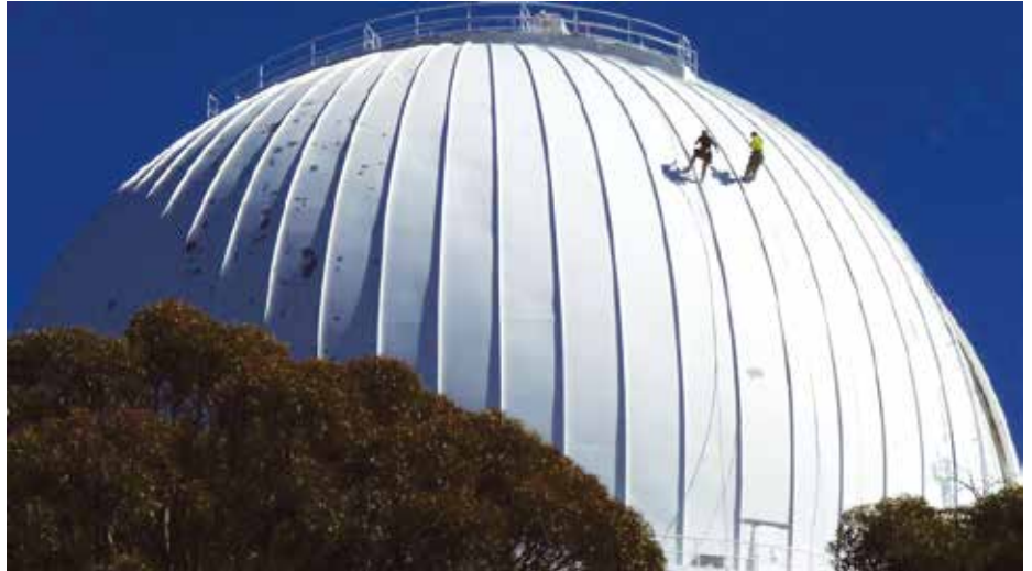
The guys from Programmed Property Services abseil down the outside of the dome, spraying paint while they go. Conveniently, the dome rotates so they can always be working in the warmth of the sun. Credit: Guy Albertson
