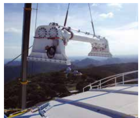
The dome shutter emergency brake before hoisting onto the top of the AAT dome. The brake itself weighs four tonnes.
