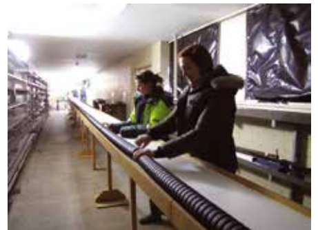
Figure 7. Carolin Barth and Sue Wilson (fibre optic assistants) inserting the cable into the Triflex conduit.
