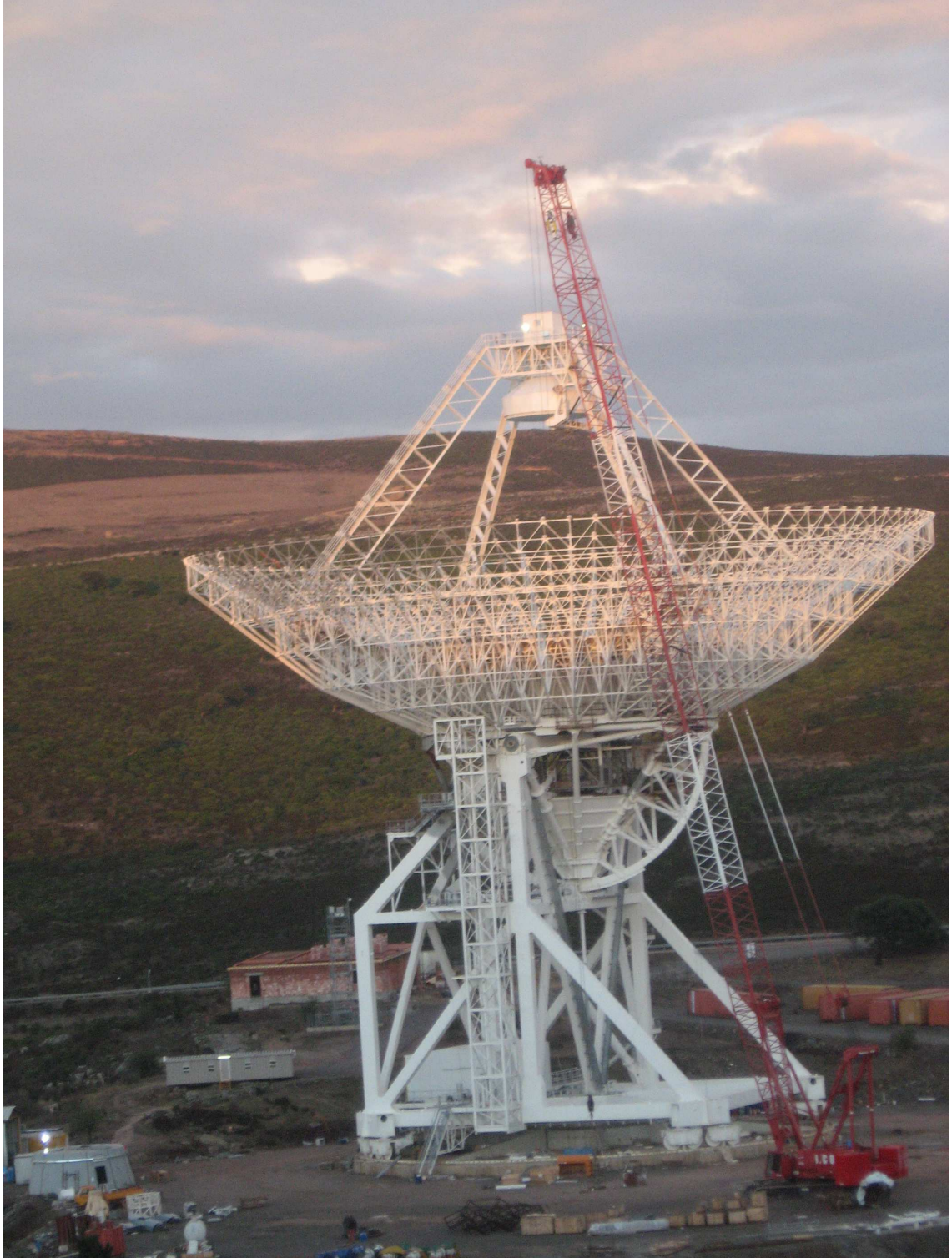
Figure 2.1 The Sardinia radio telescope under construction 35 km North of Cagliari, Sardinia, Italy. Photo Credit: T. J. Johnson
