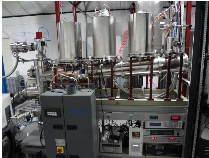
Fig.1 The Cooling Bus. In front is the getter for the recirculation - purification.
