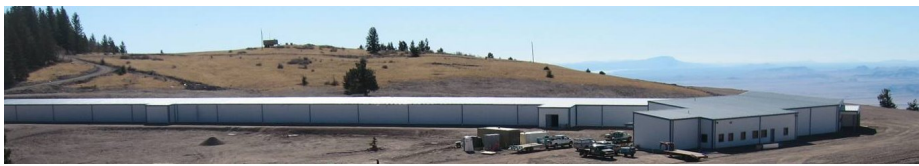
Fig. 6 A recent photograph of the MROI beam combining facility. To the left in the photograph extends the single pass delay lines in a 190m long building. To the right in the photograph is the location of the center of the array arms to be laid out in an equilateral-Y with the longest baseline attaining nearly 345m (adapted from Creech-Eakman et al, 2008).
